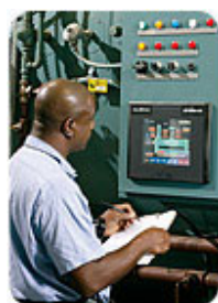
Cleaver-Brooks' Hawk ICS is a control system for boiler/burner management.
